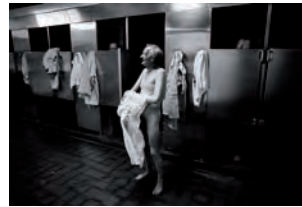
Plate 9 The shower facilities in Ozanam House. 1983.
